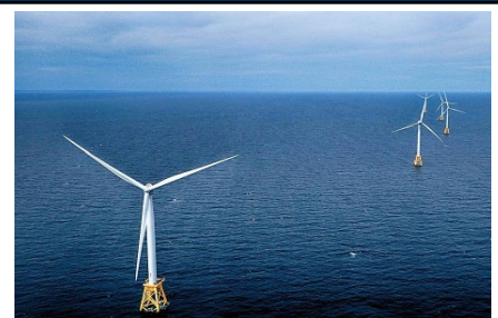
Offshore Wind Turbine
